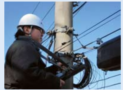
Splicing aerial drop cable
